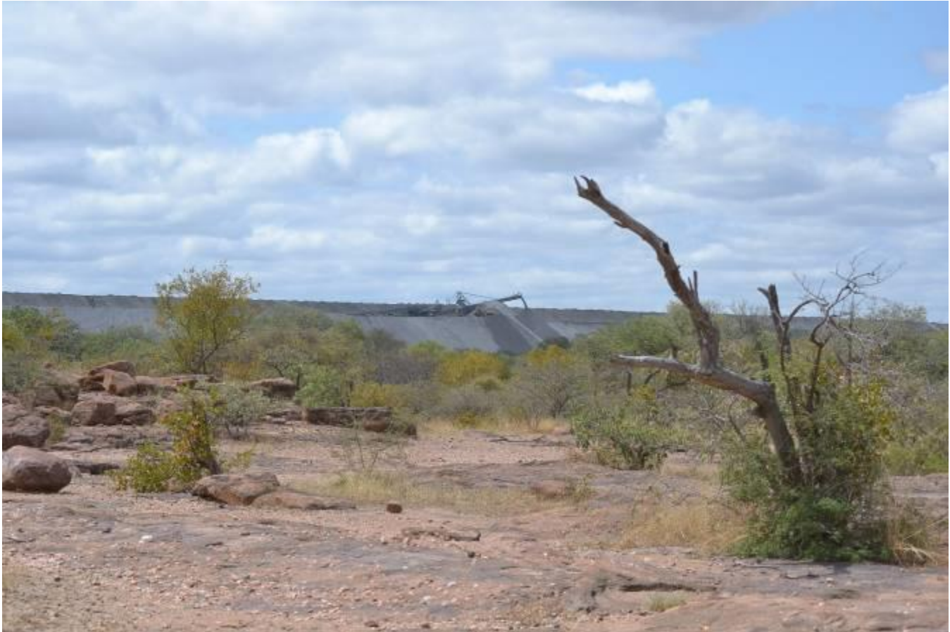
Figure 13 – The active western face of the ash dump, as viewed from the area into which the ash dump is proposed to expand
