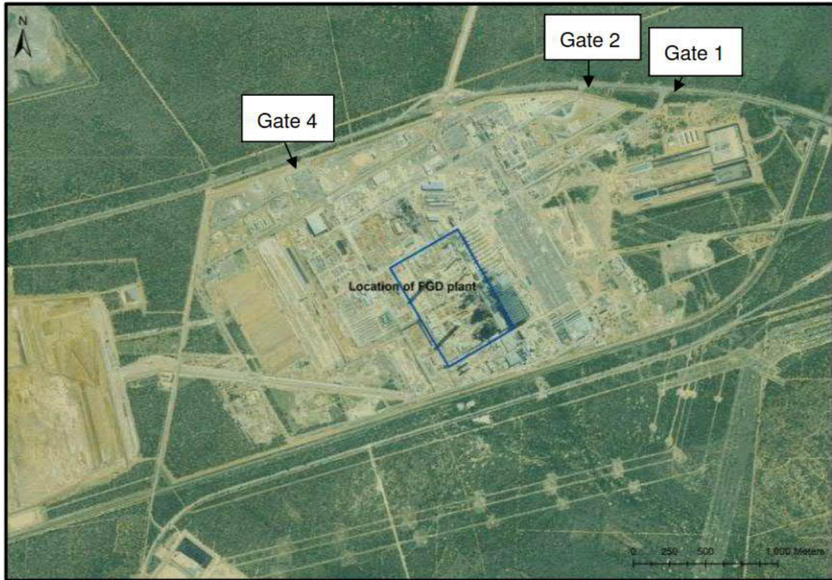
Figure 6-17: Access Gates at Medupi Power Station
