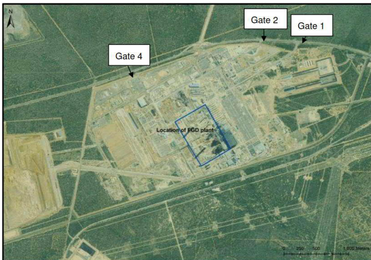
Figure 6-18: Access Gates at Medupi Power Station
