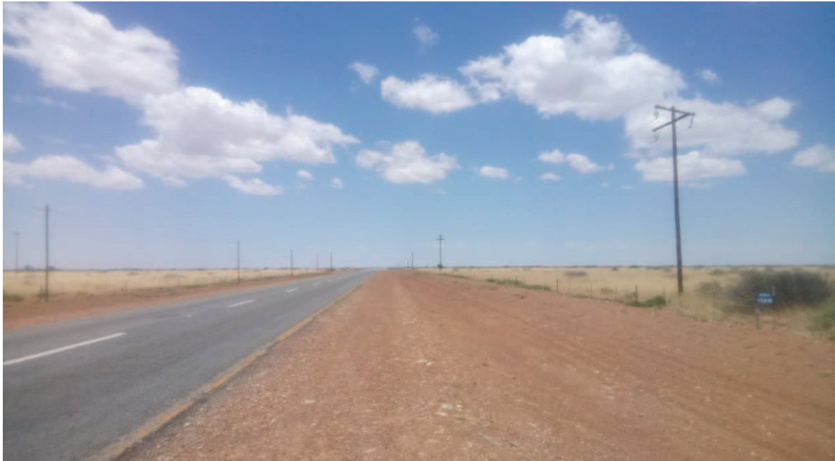
Figure 43: Existing powerlines along the N18
