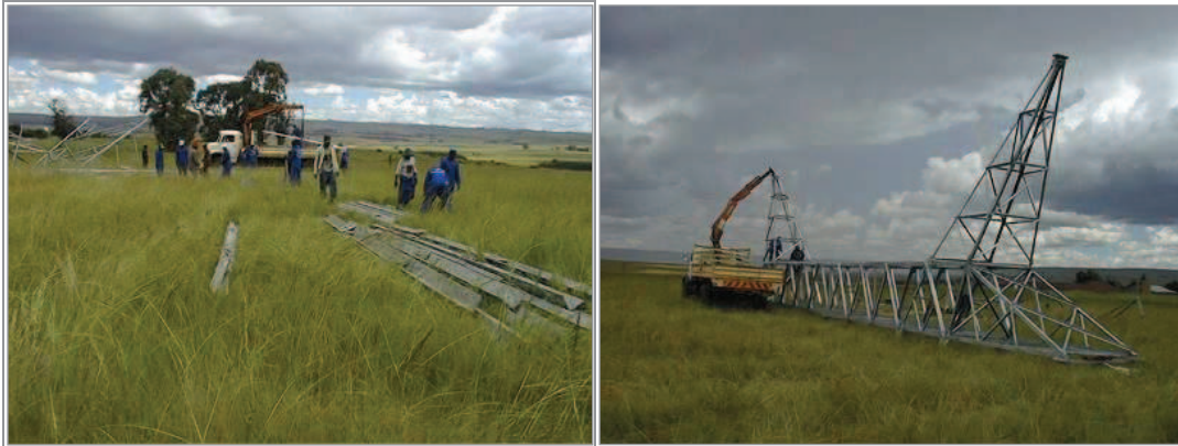
Figure 21: Delivery of steel (left) and assembly of tower (right)
