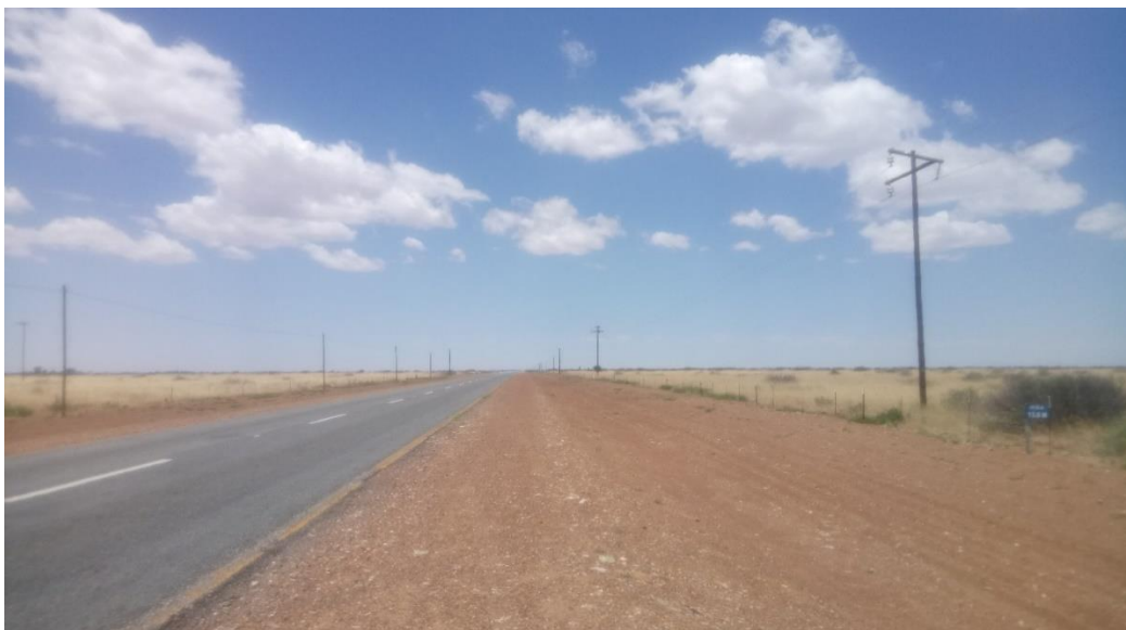
Figure 52: Existing powerlines along the N18
