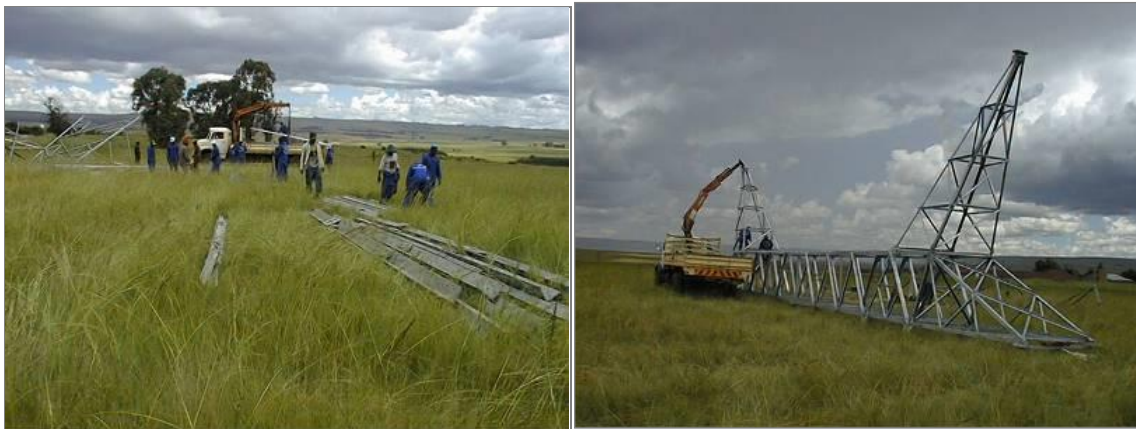
Figure 27: Delivery of steel (left) and assembly of tower (right)
