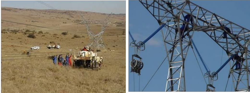
Figure 28: Stringing with pilot tractor (left) and pulleys (right)
