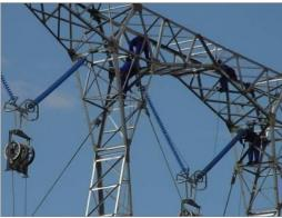
Figure 28: Stringing with pilot tractor (left) and pulleys (right)
