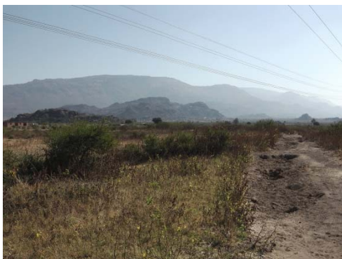
Figure 30: Corridor following the existing power line west towards the Lesideng substation.
