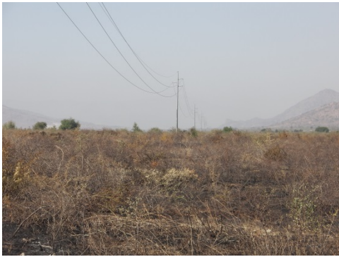
Figure 2: View of corridor following existing power line near Nkwe sub – visual impact moderate.
