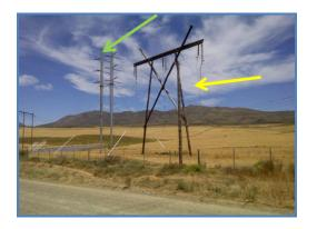
Figure 3: South – easterly view with the existing 400 kV Powerline from Proteus Substation (yellow arrow) and the 132 kV Powerline from Blanco Substation (green arrow). Both Powerlines feed into the existing Outeniqua Substation located to the left of the road.
