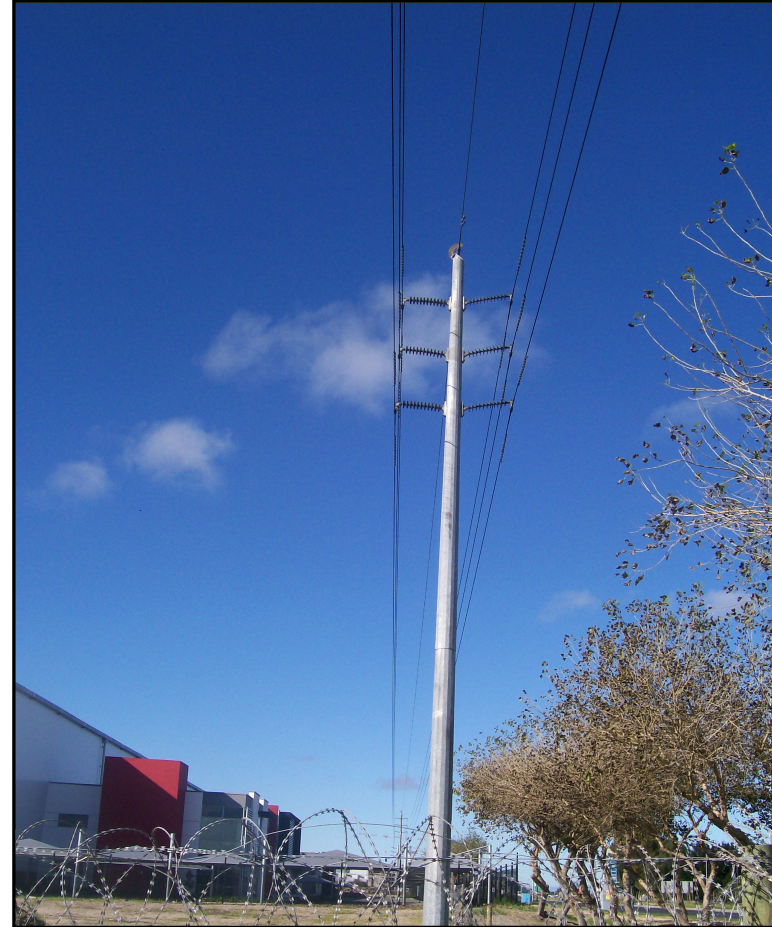
Plate 19: Example of a steel monopole structure
