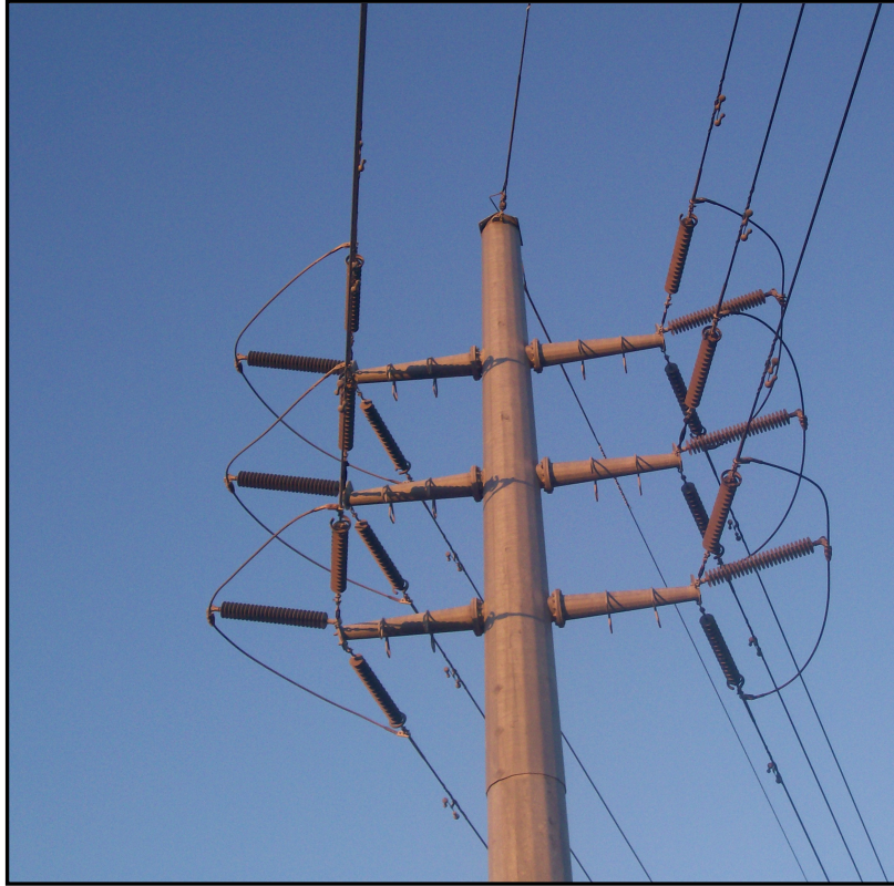
Plate18: Close-up photo of a steel monopole
