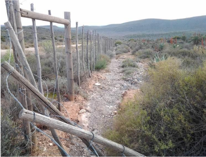
Figure 17: Some of the erosion visible in the area.
