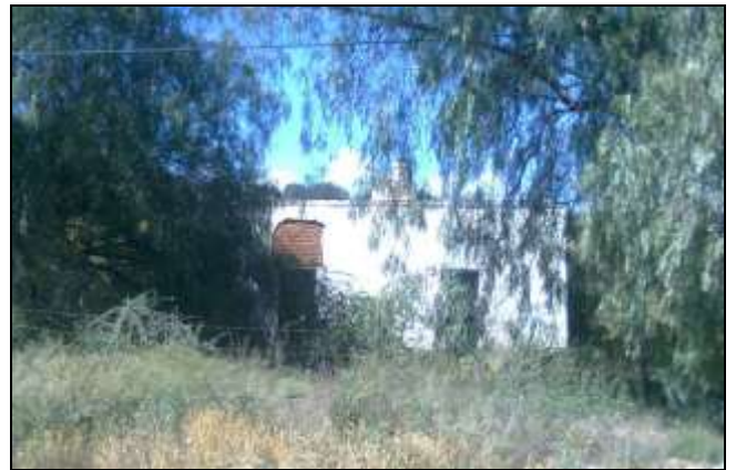
Figure 31: A flat-roofed labourers' cottage at point 049.
