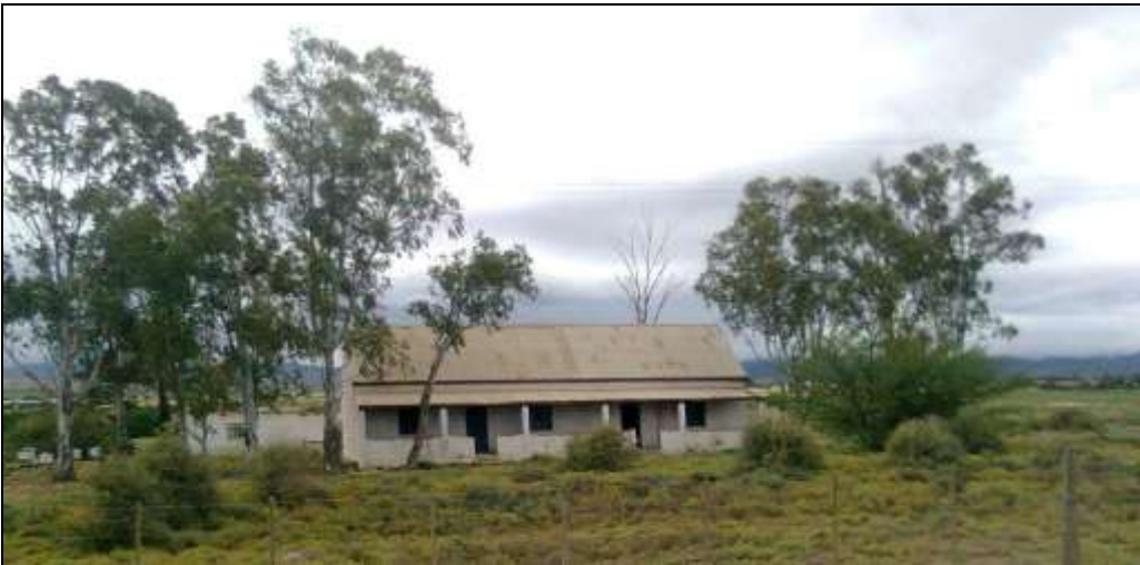
Figure 29: A vernacular stone-built farmhouse at point 043.
