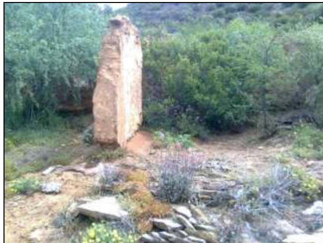
Figure 20: The central wall of the mud-brick ruin at MKR2012/002.
