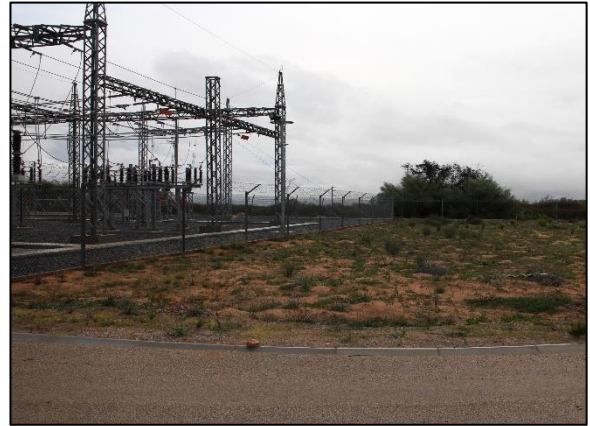
Photo 2-4: Elevated platform and barrier around the boundary of the site
