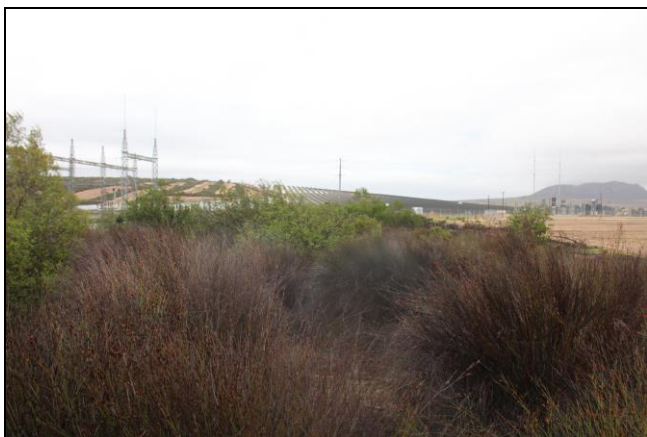
Figure 4: Strip of natural vegetation adjacent to the Substation
