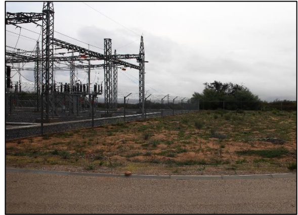
Photo 2-4: Elevated platform and barrier around the boundary of the site
