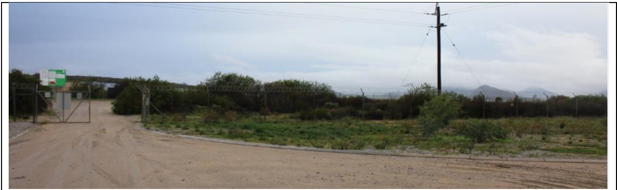
View of the access road to the east of the Paleisheuvel Substation
