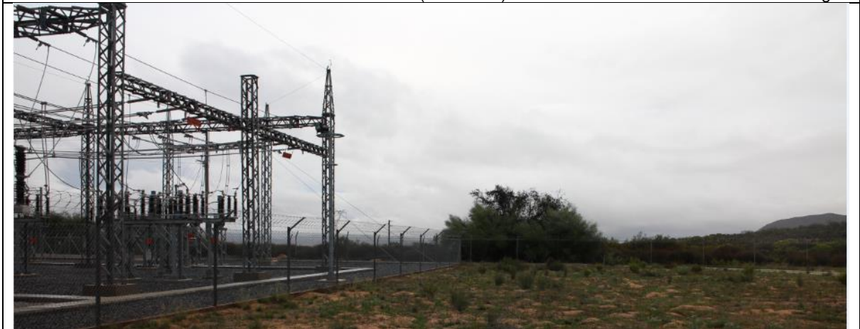
View of the area to the west of the Paleisheuwel Substation looking south
