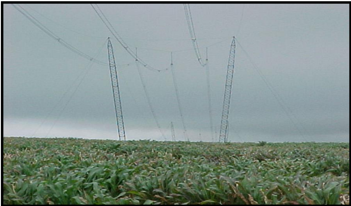
Figure 10: Cross Rope Structure
