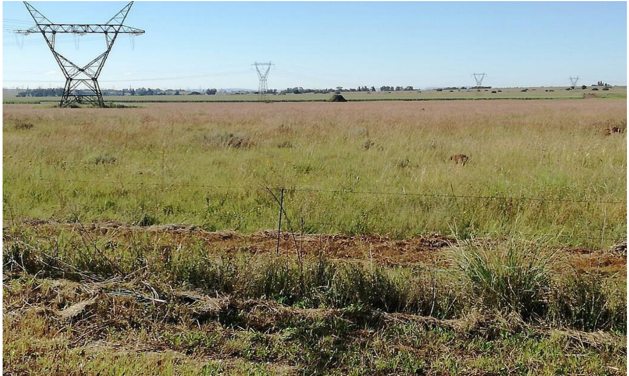
Figure 113: View of existing Powerline from Pluto substation to Watershed substation
