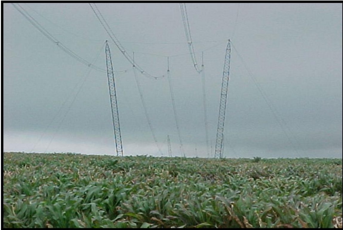
Figure 10: Cross Rope Structure
