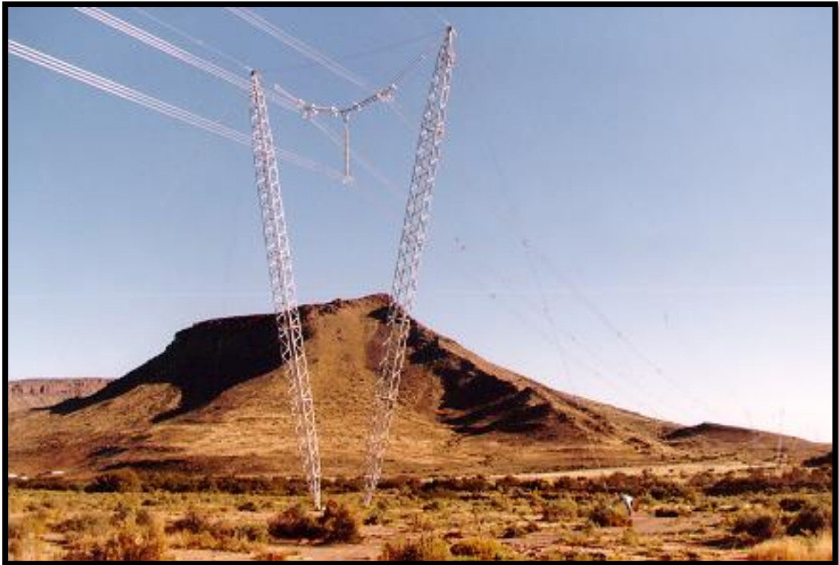
Figure 8: Guyed V structure
