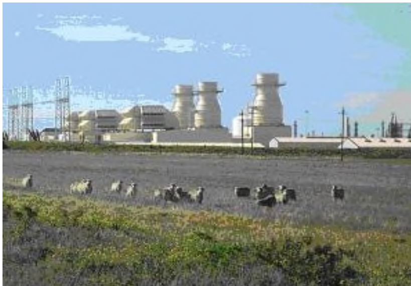
Plate 2: An existing Gas Turbine Power Station (Gourikwa) as seen from within 1km. The image highlights that the main visual mass is provided by the medium high structures that combine to provide the main visual bulk.
