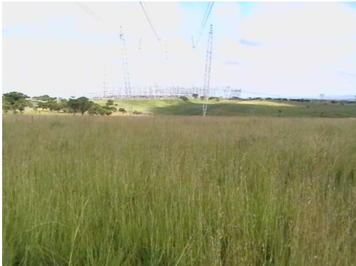
Cross-roped suspension tower
