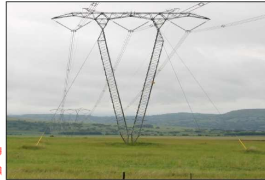
Guyed-V suspension tower
