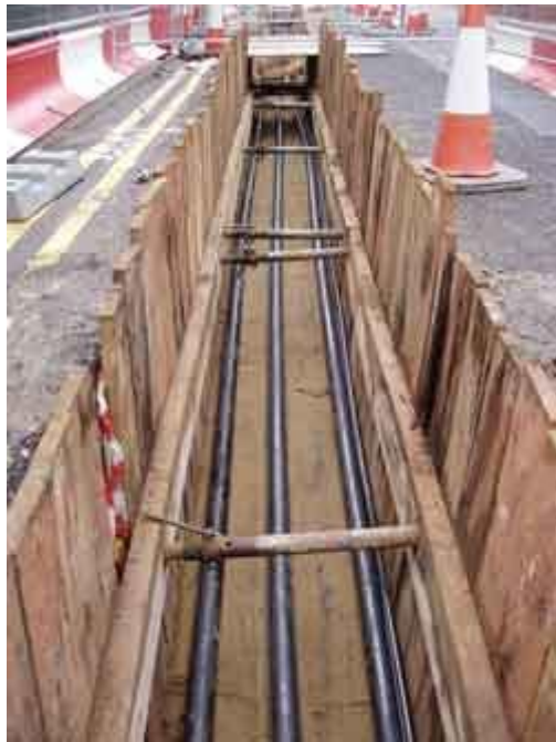
Figure F-1: Direct buried cable being installed [2].
