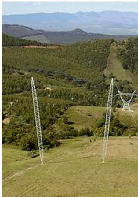
Figure A-7: Tower Type 529 (Cross-Rope).
