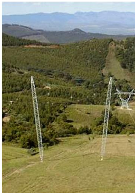
Figure A-2: Tower Type 524 (Cross Rope).
