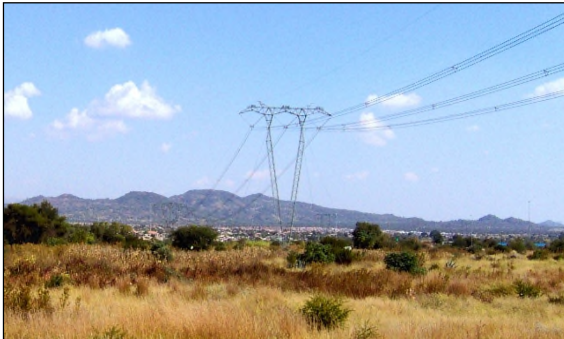
Figure 2.4: Compact Cross-roped suspension tower
