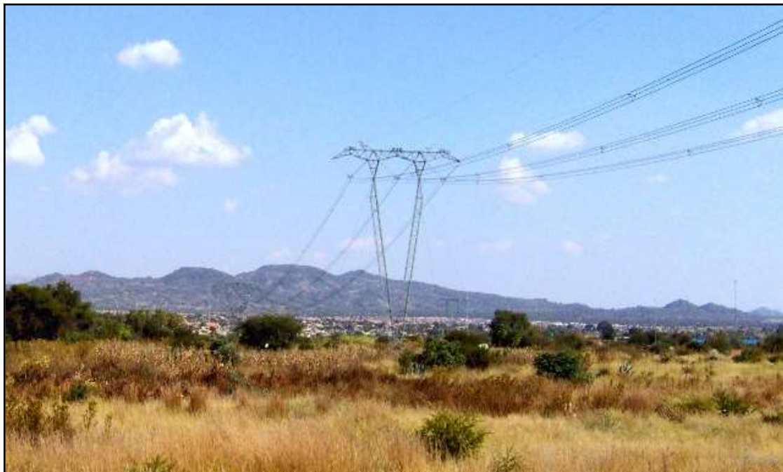
Figure 2.3: Compact Cross-roped suspension tower
