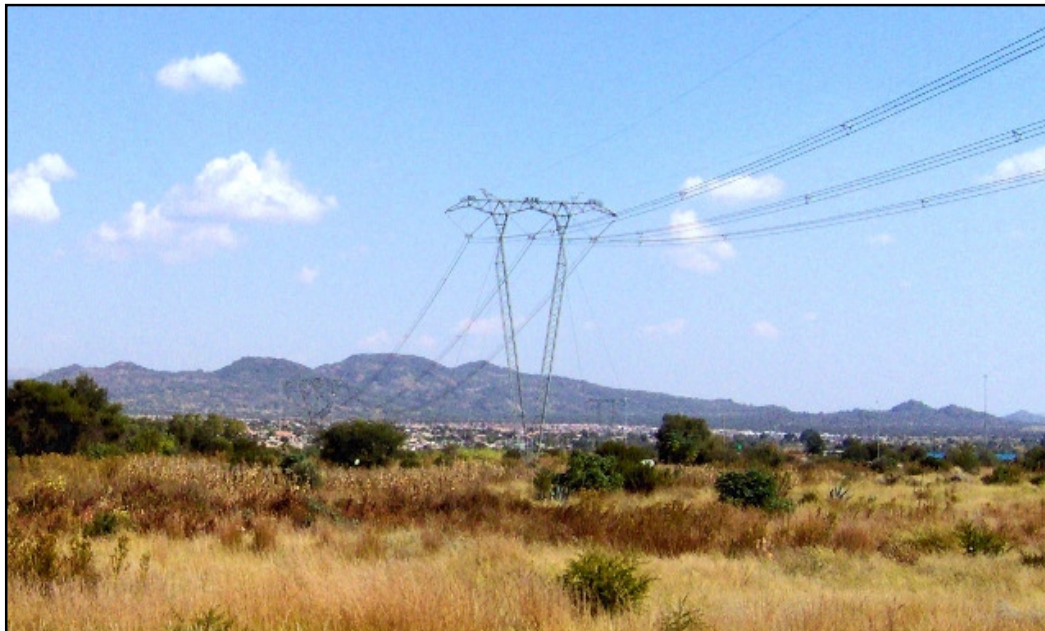
Figure 2.3: Compact Cross-roped suspension tower
