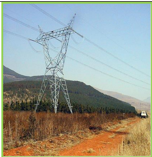
Figure 15: Photographic Self-supporting suspension tower.
