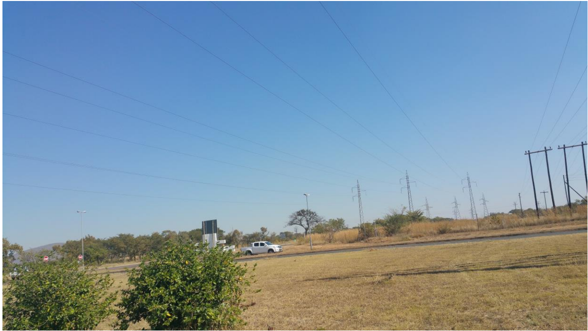
Photo ii: the photo showing the crossing of the road from Groblersdal Substation
