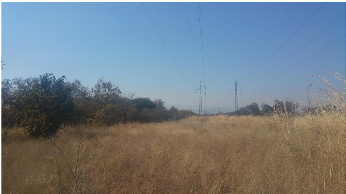
Fig v: The proposed 132kV will run on the left hand side of the existing power line
