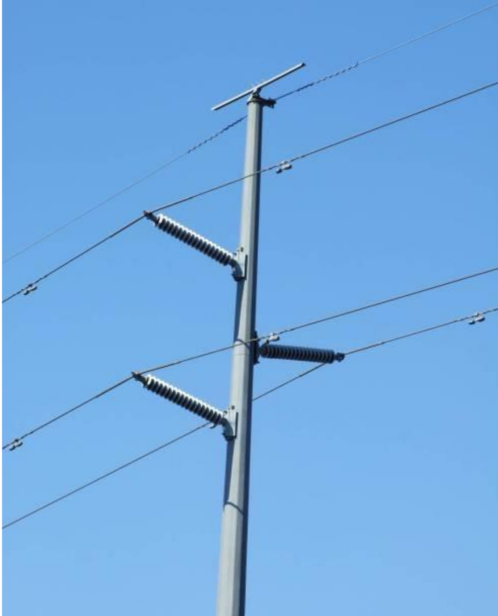
Figure 10: Example of steel monopole structure to be used. The full illustrative details has been included under Appendix c
