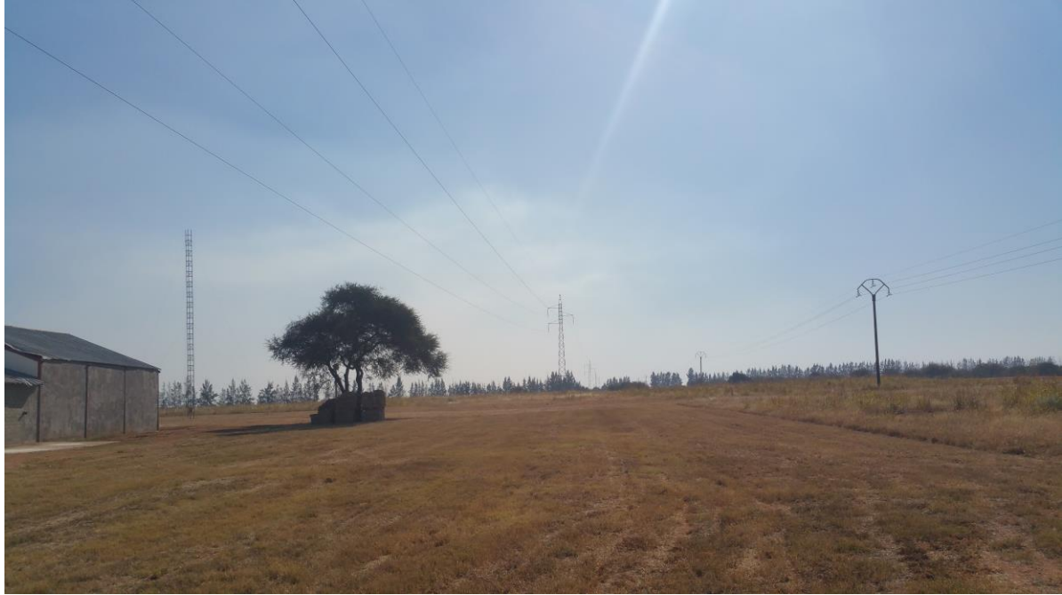
Figure viii: showing the near tear off position
