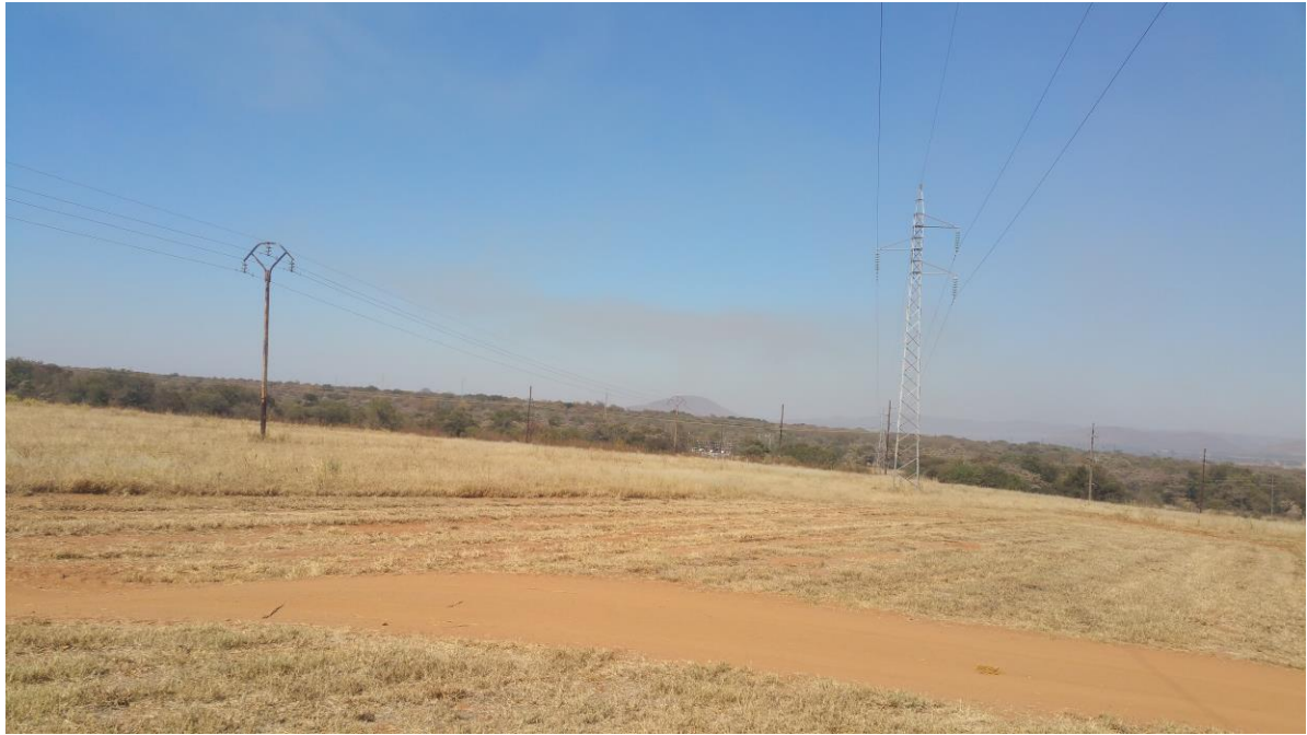
Fig iv: Showing the vacant servitude and two existing power lines i.e 22kV
