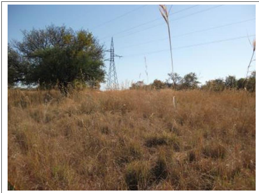
Figure 6- The second and third stretches of the proposed new power line runs across relatively pristine veld on Klipbank 26JS before entering the switching station where the last stretch of the power line will bend to the north (above).
