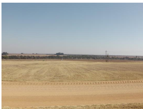
Figure 8: View near the T-off point.
