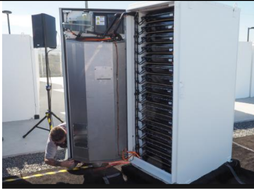
Figure 2-1: Battery cells in a battery module
