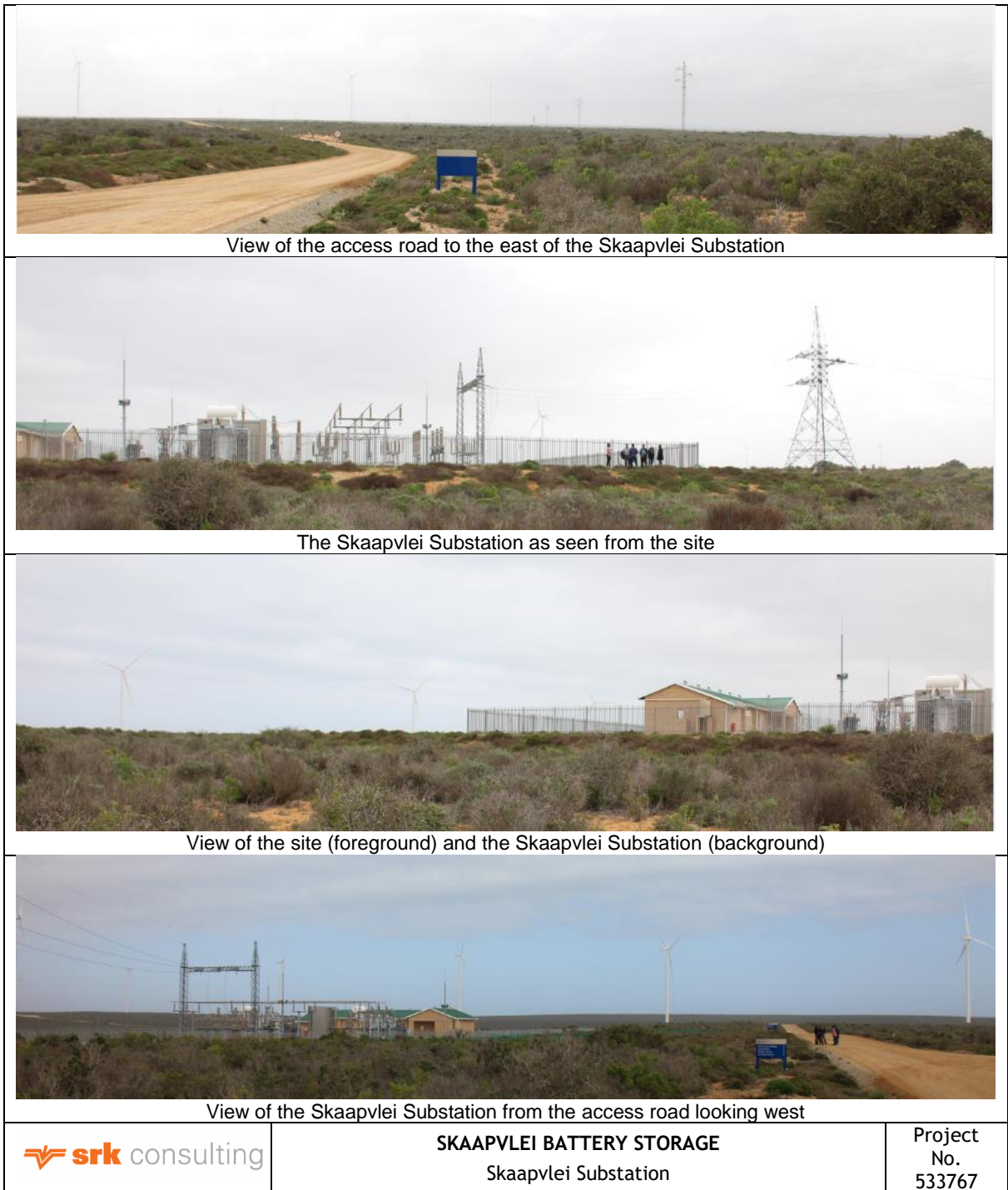
Figure 3-2: The Skaapvlei Substation and proposed site
