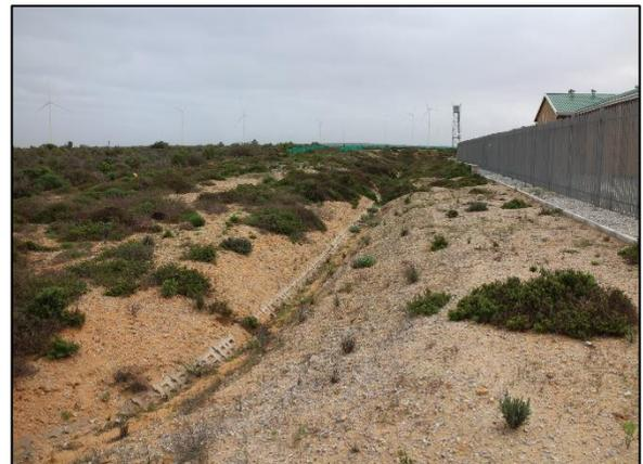
**Photo 2-4: Excavated trench around the boundary of the site**
