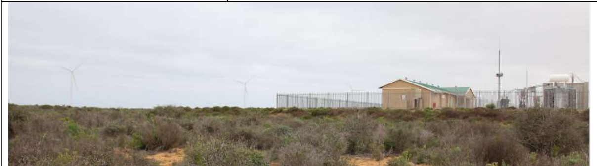
View of the site (foreground) and the Skaapvlei Substation (background)
