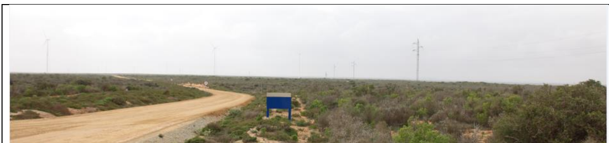
View of the access road to the east of the Skaapvlei Substation
