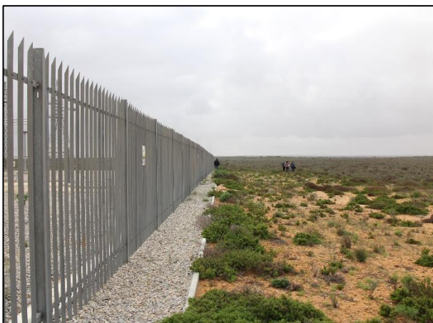
Photo 2-1: Sandy soils with revegetated areas around the site. Shallow sloping and predominantly brush vegetation
