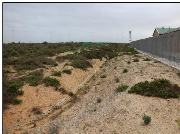
Photo 2-4: Excavated trench around the boundary of the site
