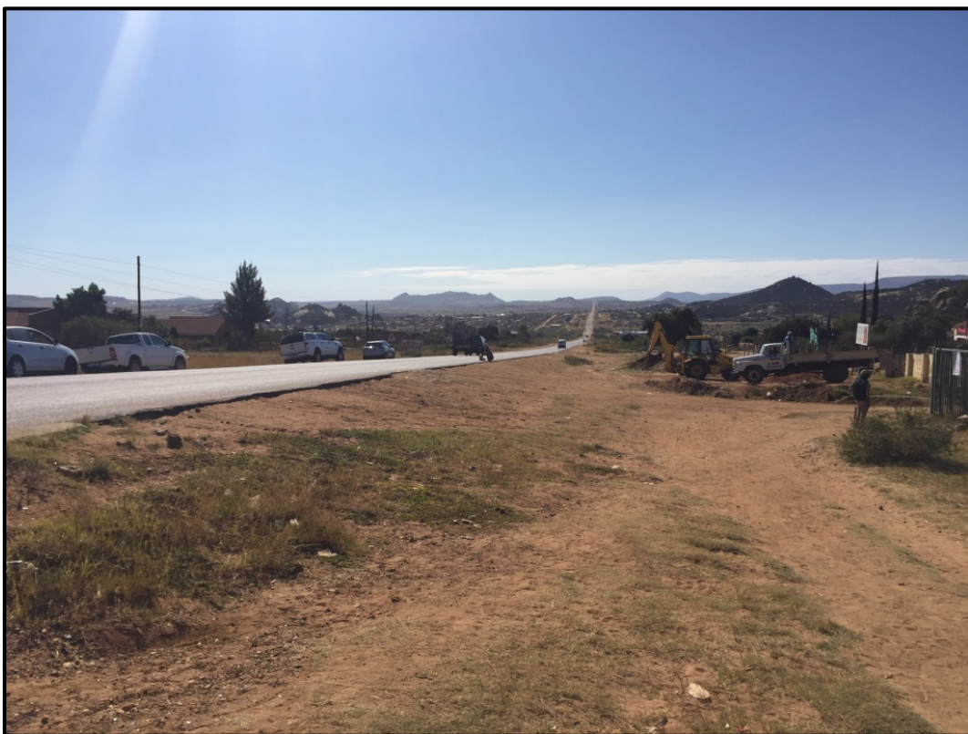
Photo 4: Syferkuil-Rampheri line route in Mankweng. University Road looking east
