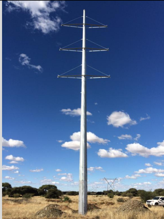
Photo plate 1: Double Circuit monopole structures
