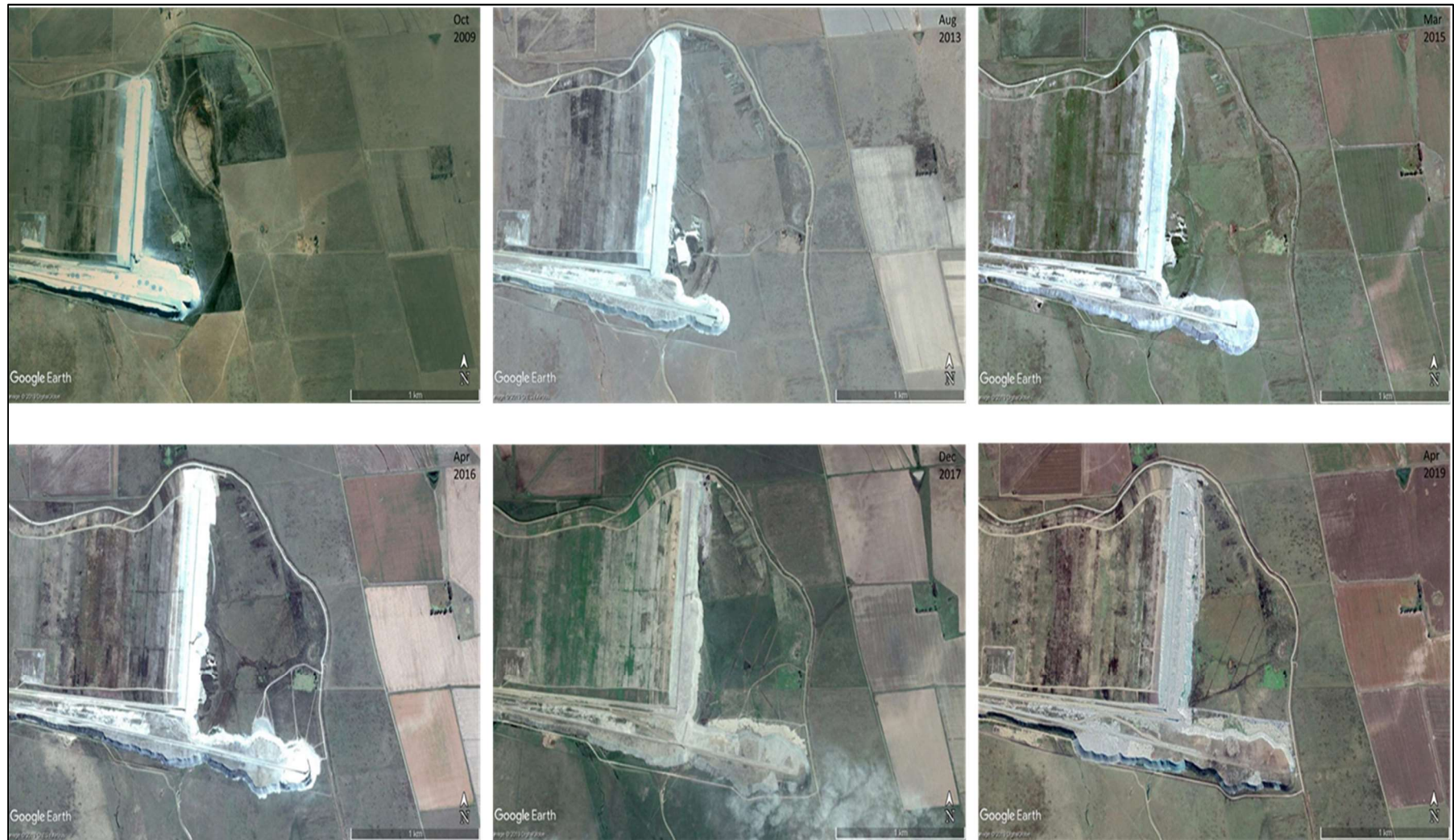
Figure 5.2: Historical aerial images of the ADF showing the advancement between October 2009 and April 2019.
