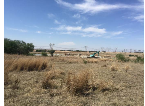
Photo 4. Cleaning in progress at PMD17
