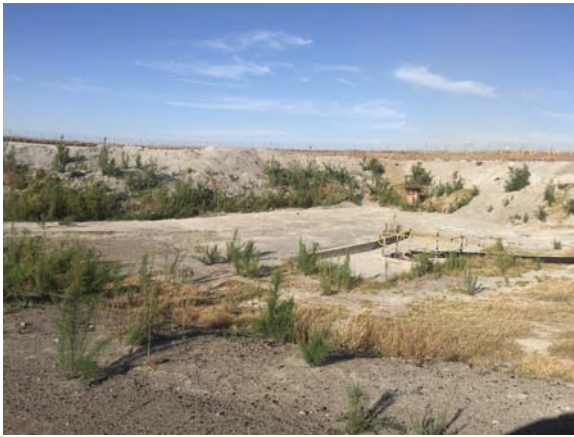
Photo 1 General site conditions
