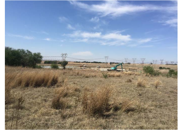
Photo 4. Cleaning in progress at PMD17
