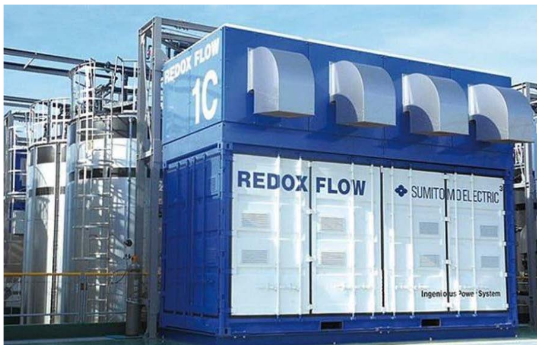
Figure 20: Redox Flow BESS equipment
