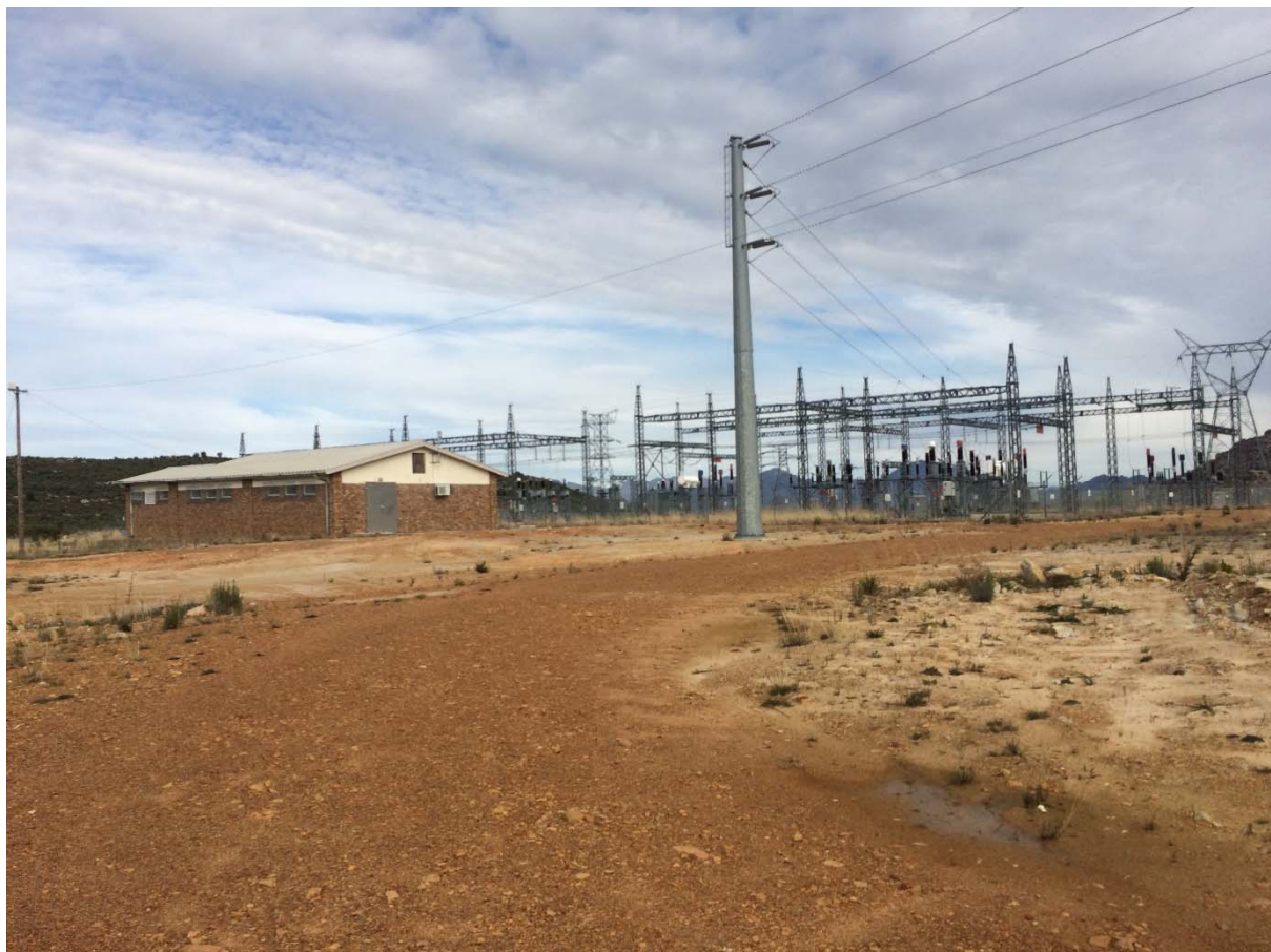
Figure 1: Cleared area within the Witzenberg Substation proposed for BESS footprint
