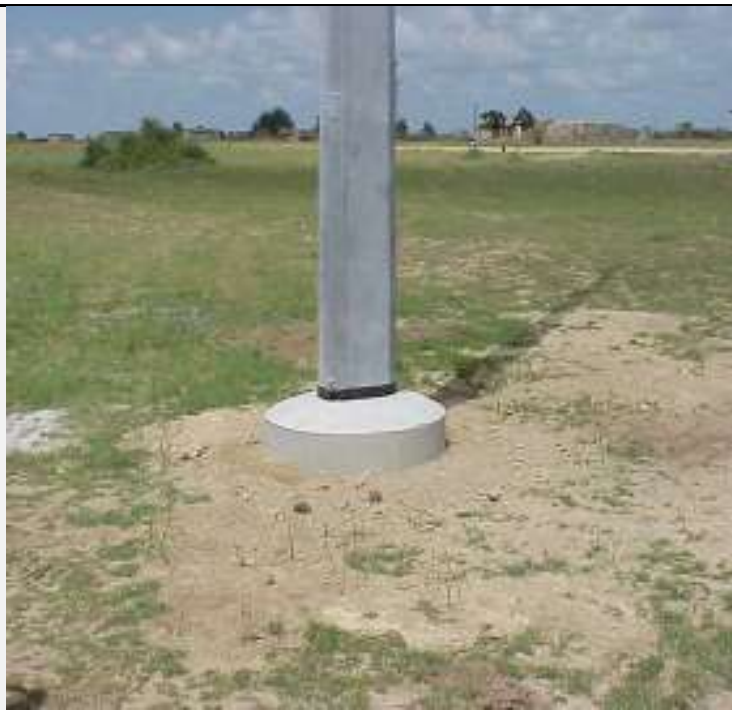
Figure 3: Single circuit steel mono-pole structures to be used for the Pylon structures
