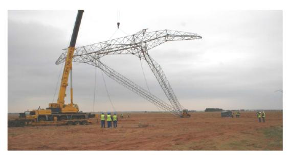
Figure 10. During construction of new infrastructure (Gyed V-pylons)<sup>10</sup>
