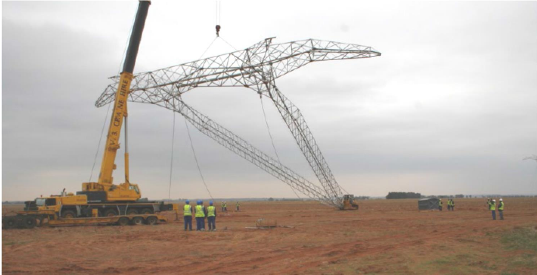
Figure 43. During construction of new infrastructure (Gyed V-pylons) 23
