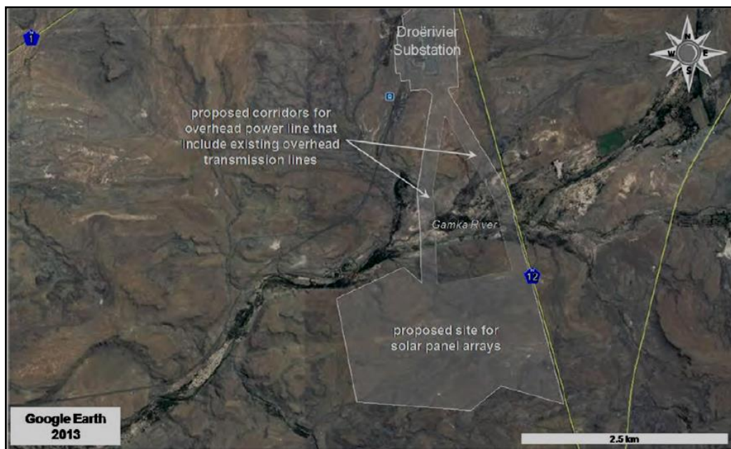
Figure 23. Proposed Solar Farm to the south of Droërivier Substation
