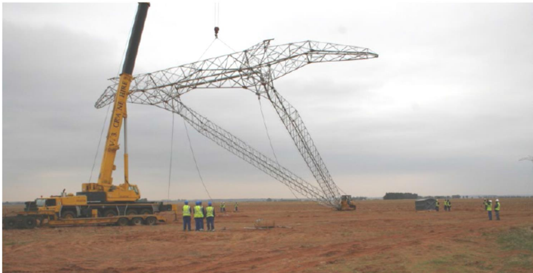
Figure 43. During construction of new infrastructure (Gyed V-pylons) 23
