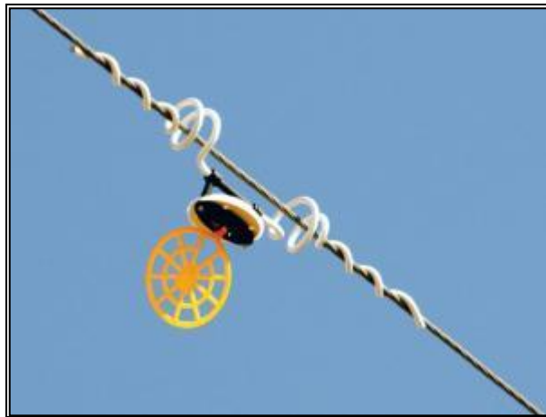
Figure 38. Bird flappers proposed as mitigation measures
