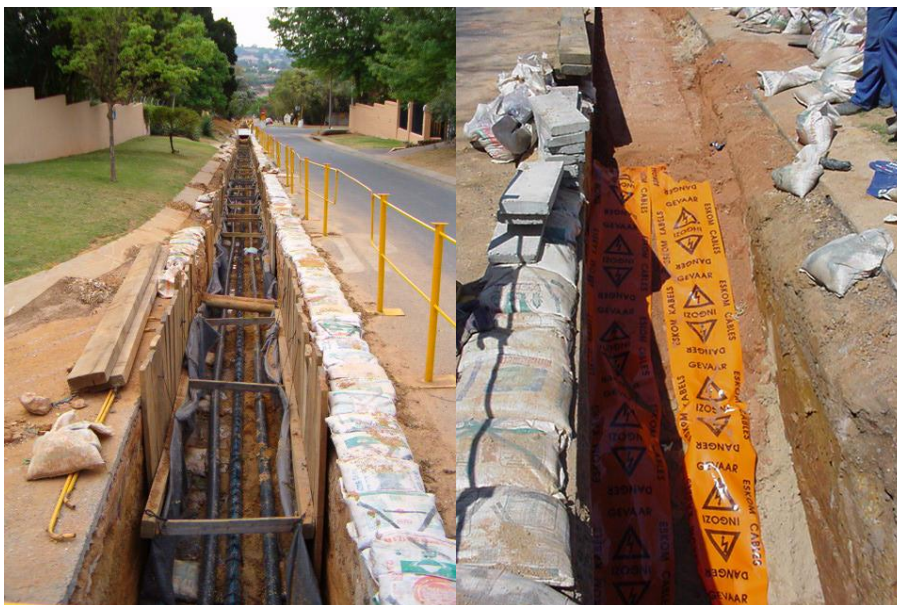
Figure 2: Cable Trenching
