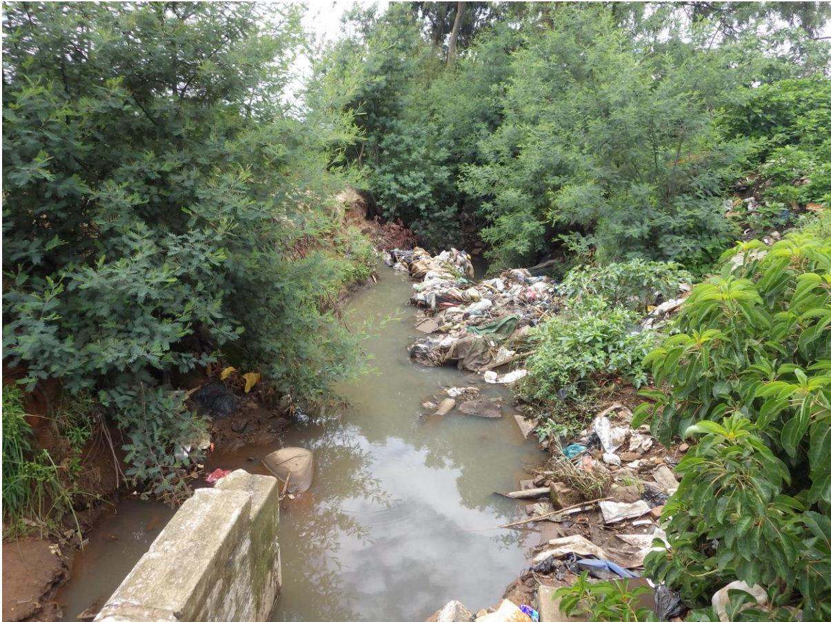
Figure 5.6 b: Solid Waste and Sewage Observed at C8 (December 2017)
