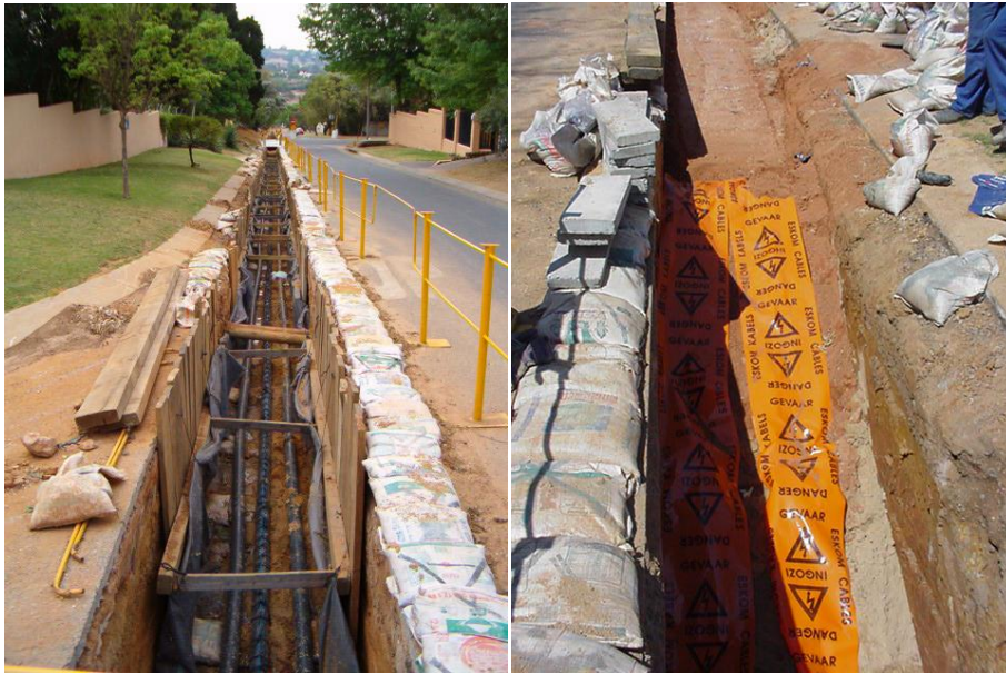
Figure 2.1: Cable Trenching
