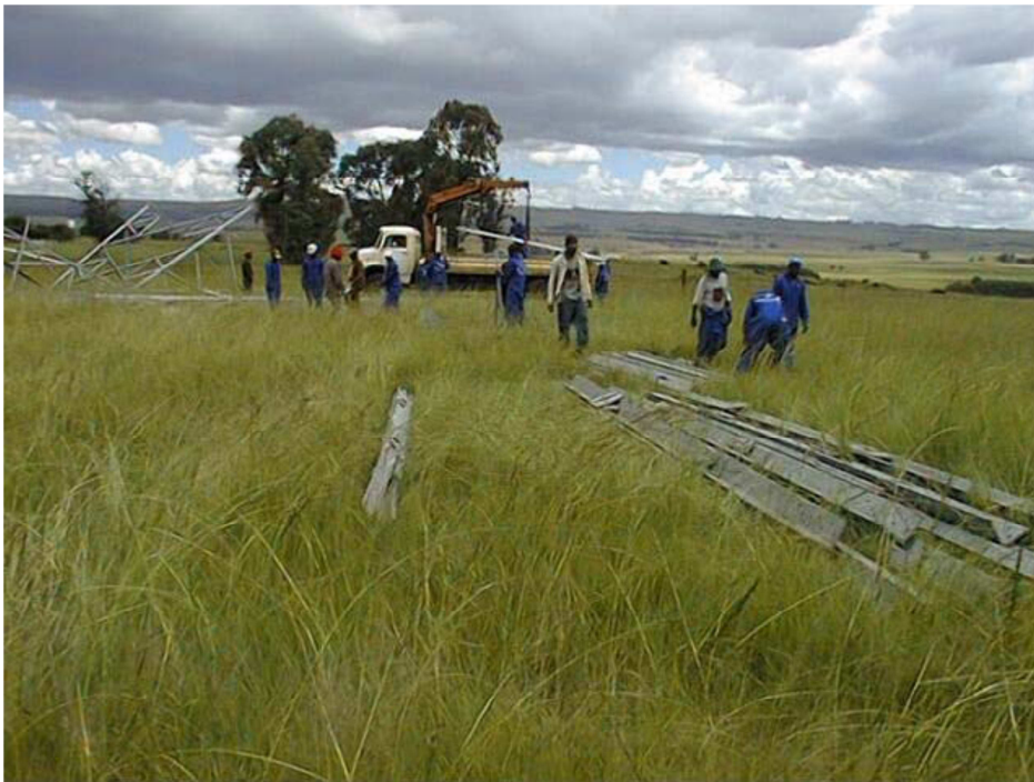
Photograph 3-4: Towers are erected on-site
