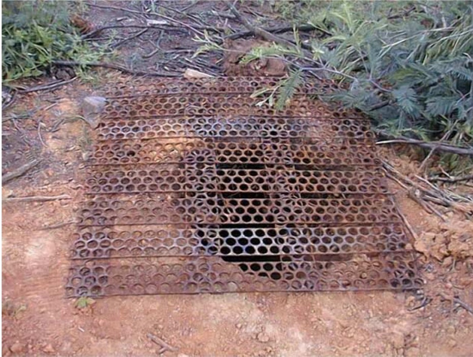
Photograph 3-3: Cover over foundations
