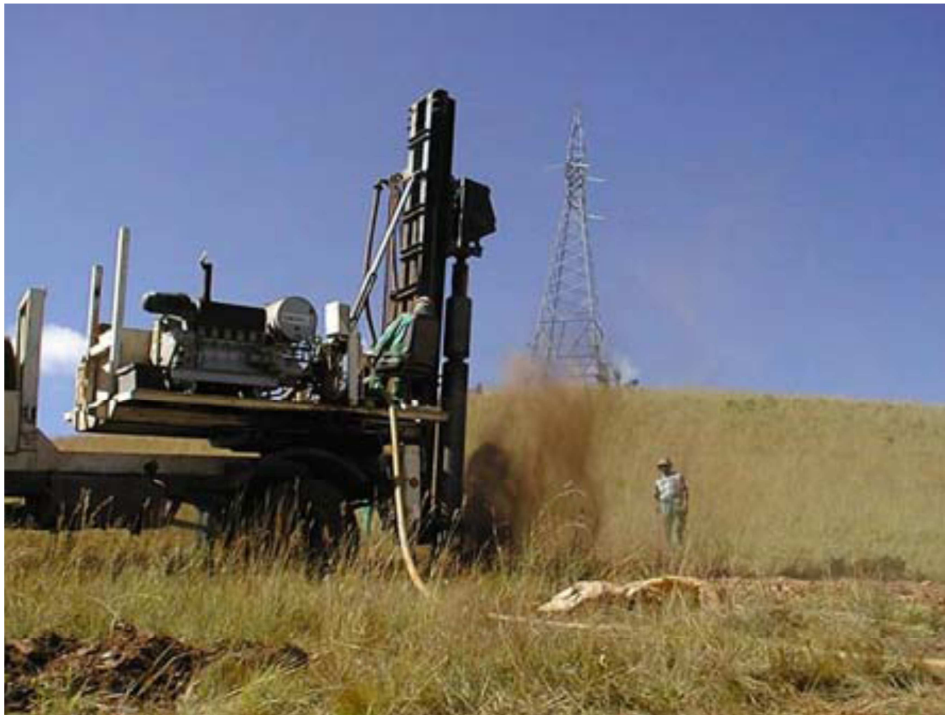
Photograph 3-2: Drilling of foundations
