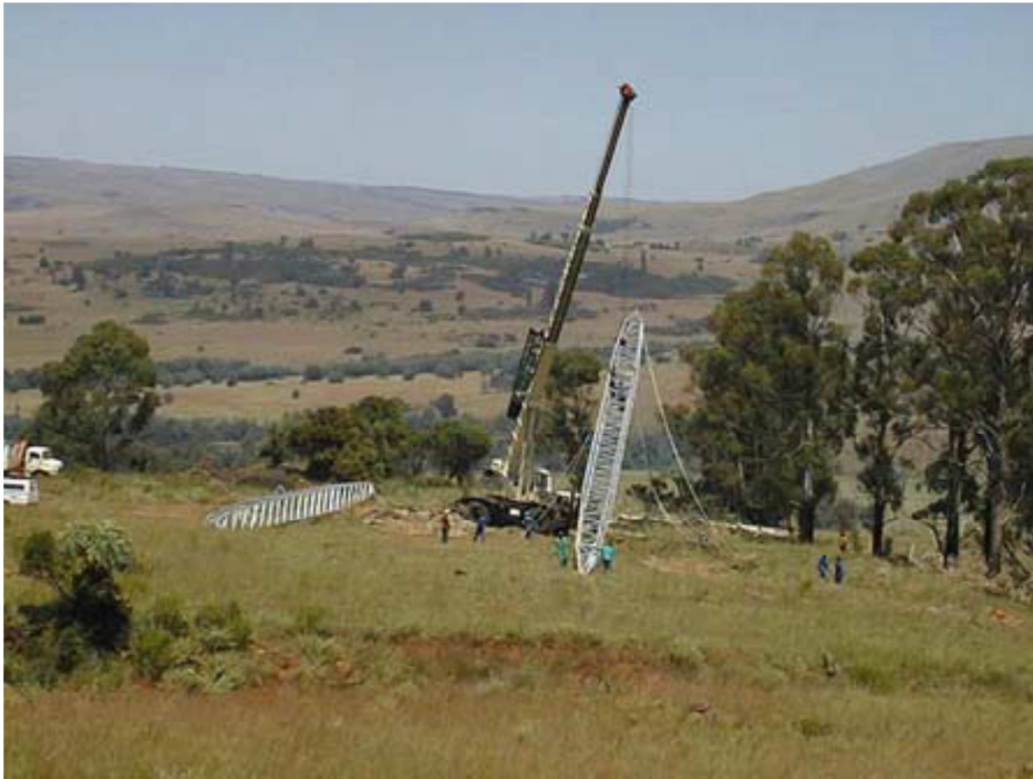
Photograph 3-5: Erection of towers by crane
