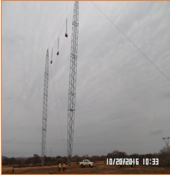
Figure 3-6: Cross Rope Suspension Tower
