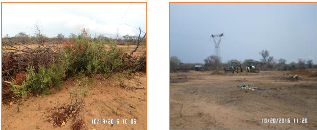
Figure 3-10: Example of clearing at tower sites
