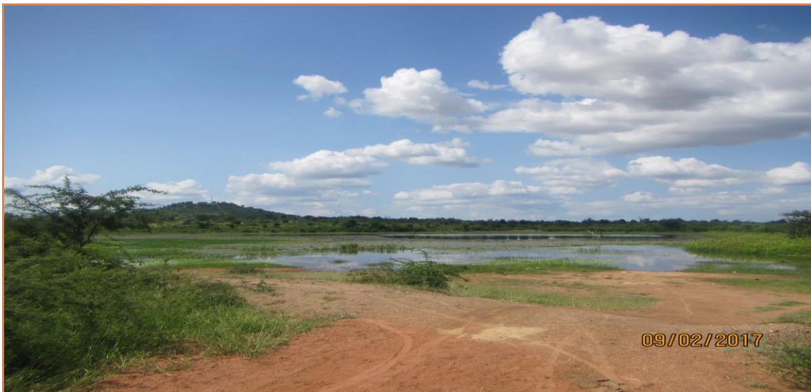
Figure 5-2: Dam near Xihoko
