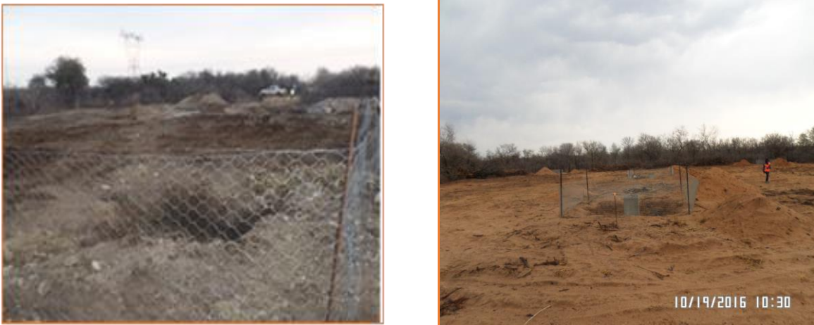
Figure 3-11: Example of excavated pits
