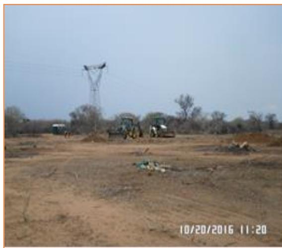
**Figure 3-9:** Example of clearing at tower sites
