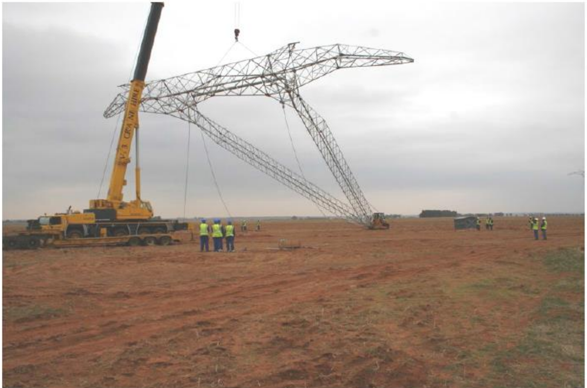
Figure 30. During construction of new infrastructure (Gyed V-pylons) 9
