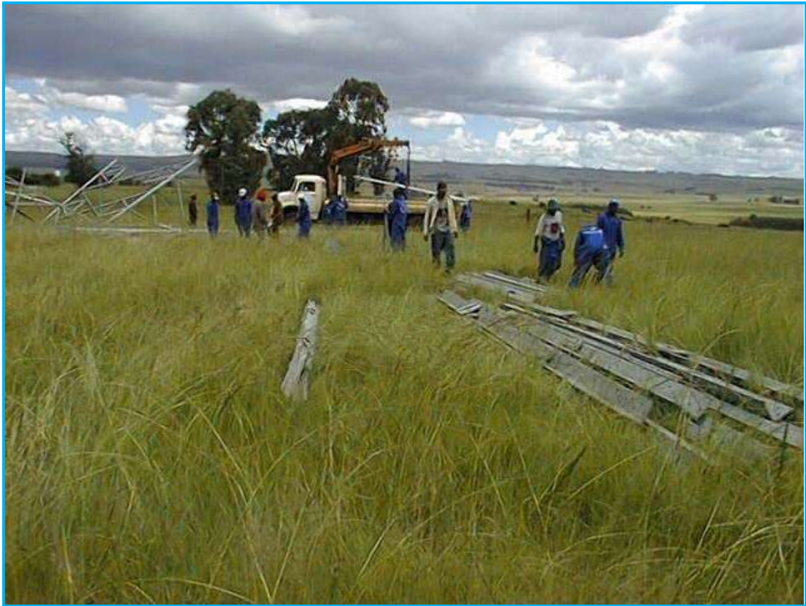
Figure 3-14: On-site erection of towers
