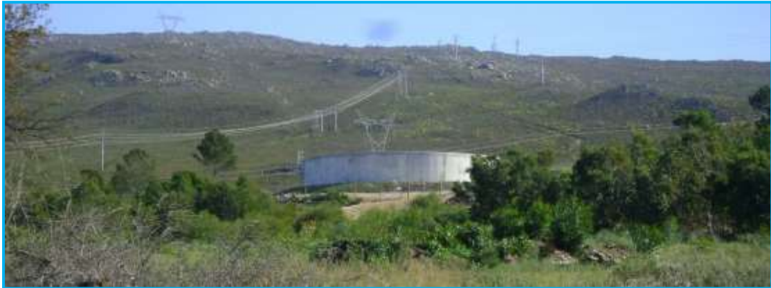
Figure 7-12: View of existing power lines on northern edge of LILO 1 corridor, with LILO 2 and LILO 3 corridors below the reservoir
