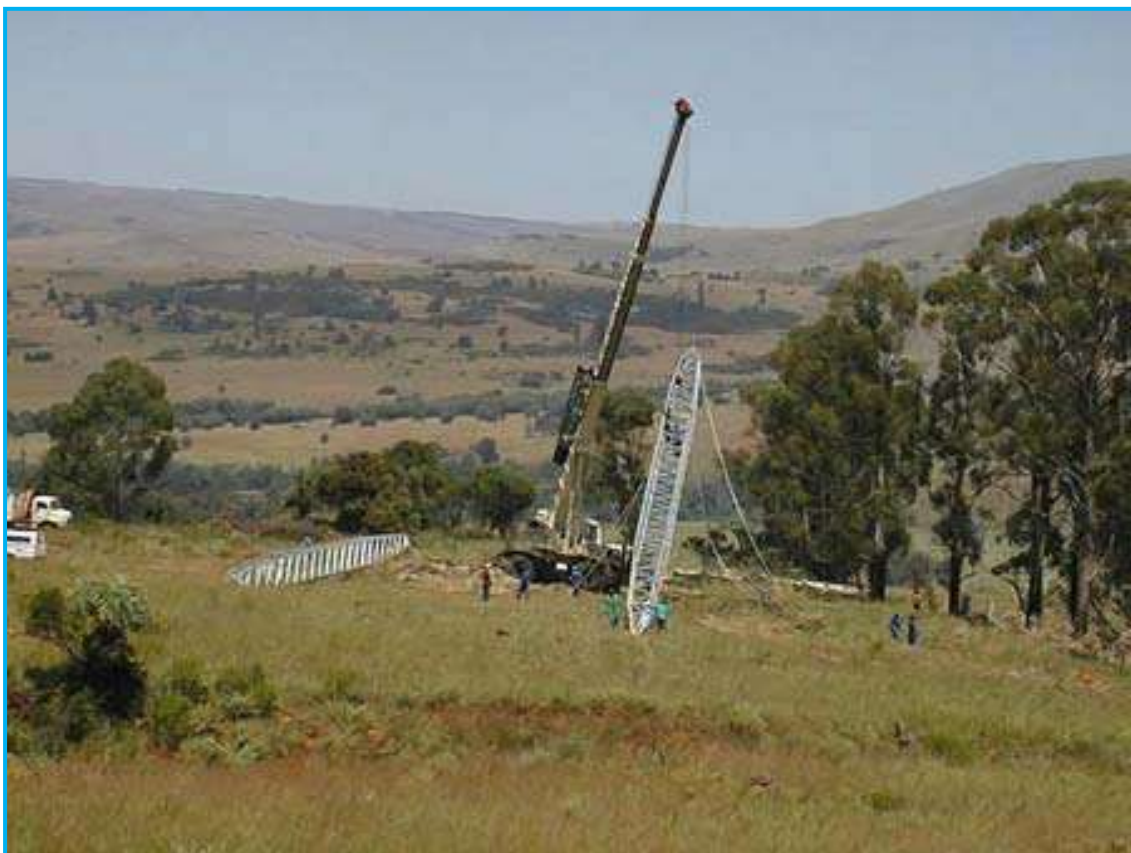
Figure 3-15: Erection of towers by crane
