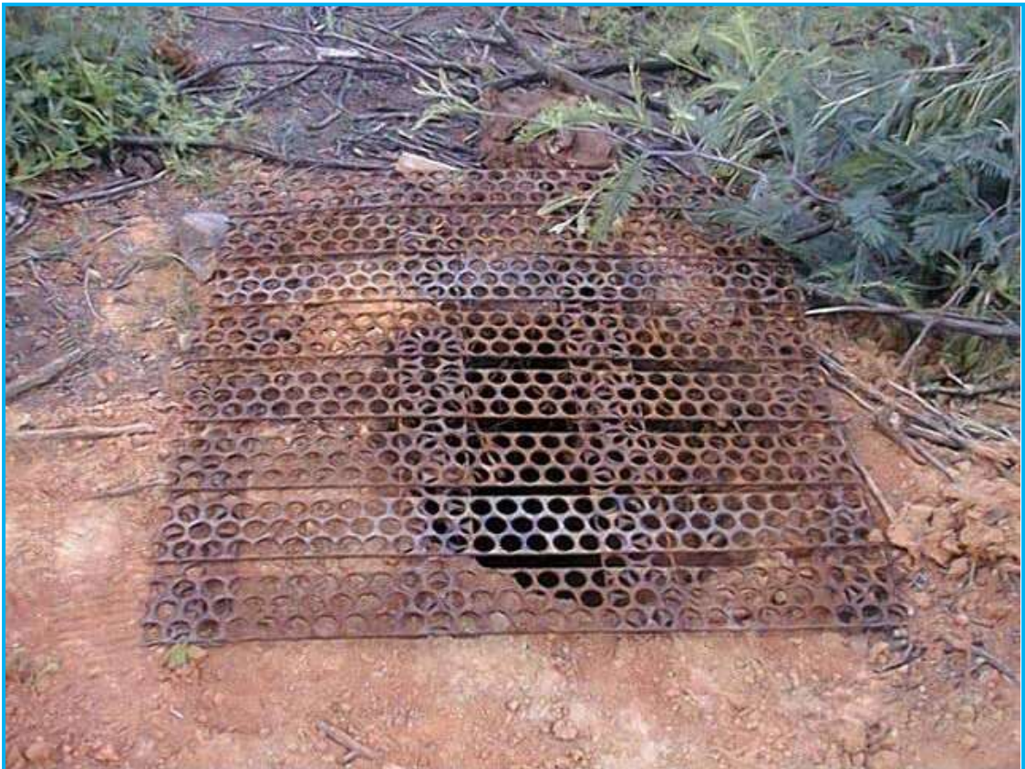
Figure 3-13: Cover for foundations
