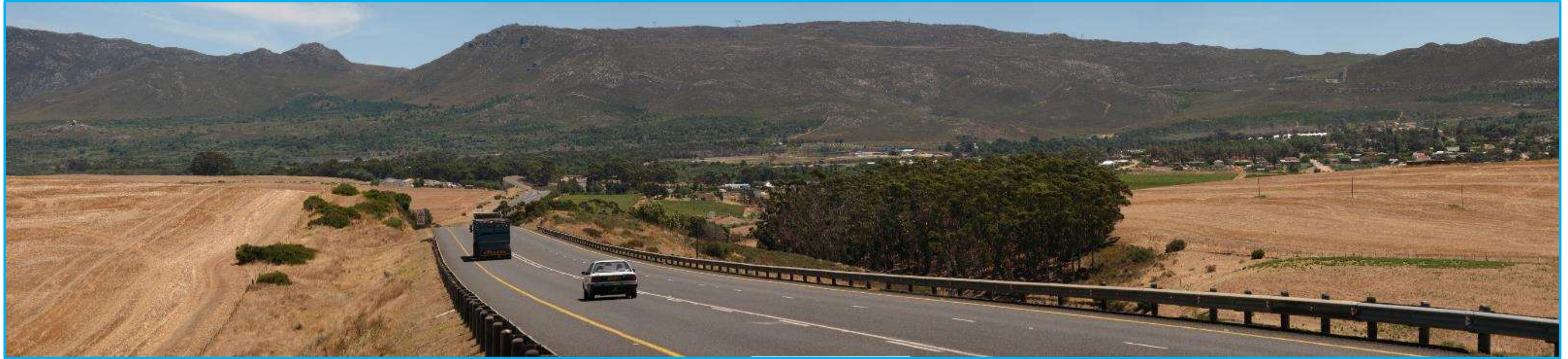
Existing view from N2 Highway Westbound
