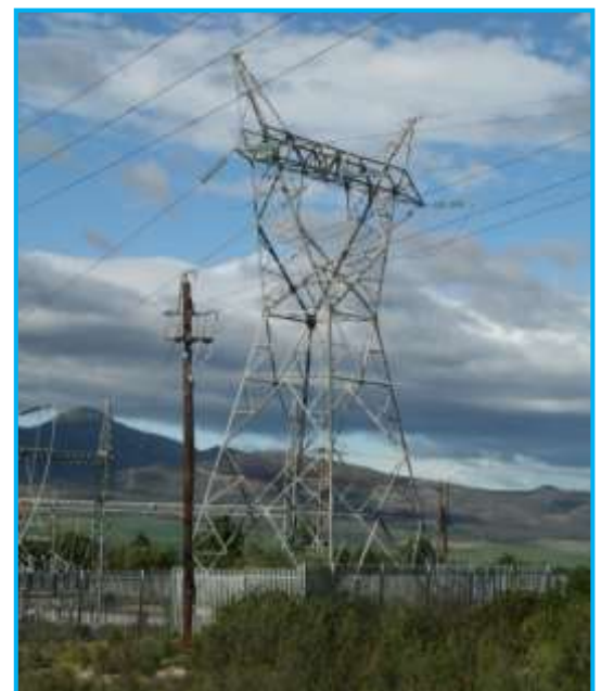
Figure 3-3: Self-Supporting Pylon
